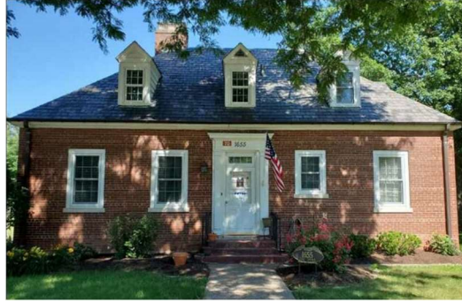
Built in 1934, Building 70 Quarters 23
